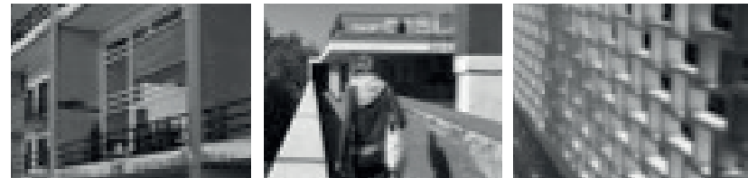
Fig. 8: Function value of ANK2 a) windows for lighting and ventilation and aesthetic b) usable terrace c) fixed shading devices.
