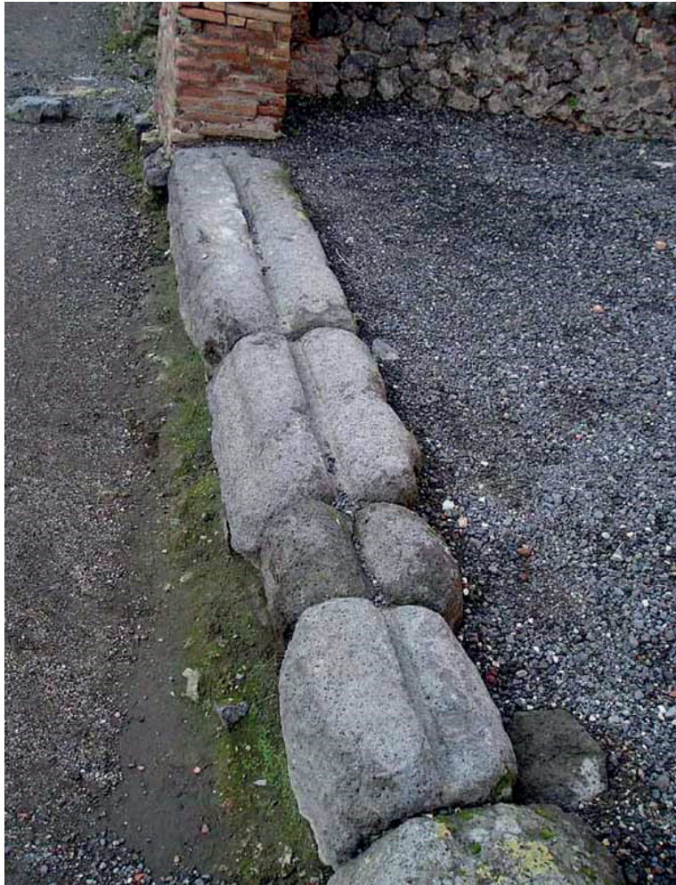
Fig. 9: Sliding door tracks at the entrance of a Roman shop in Pompeii.
