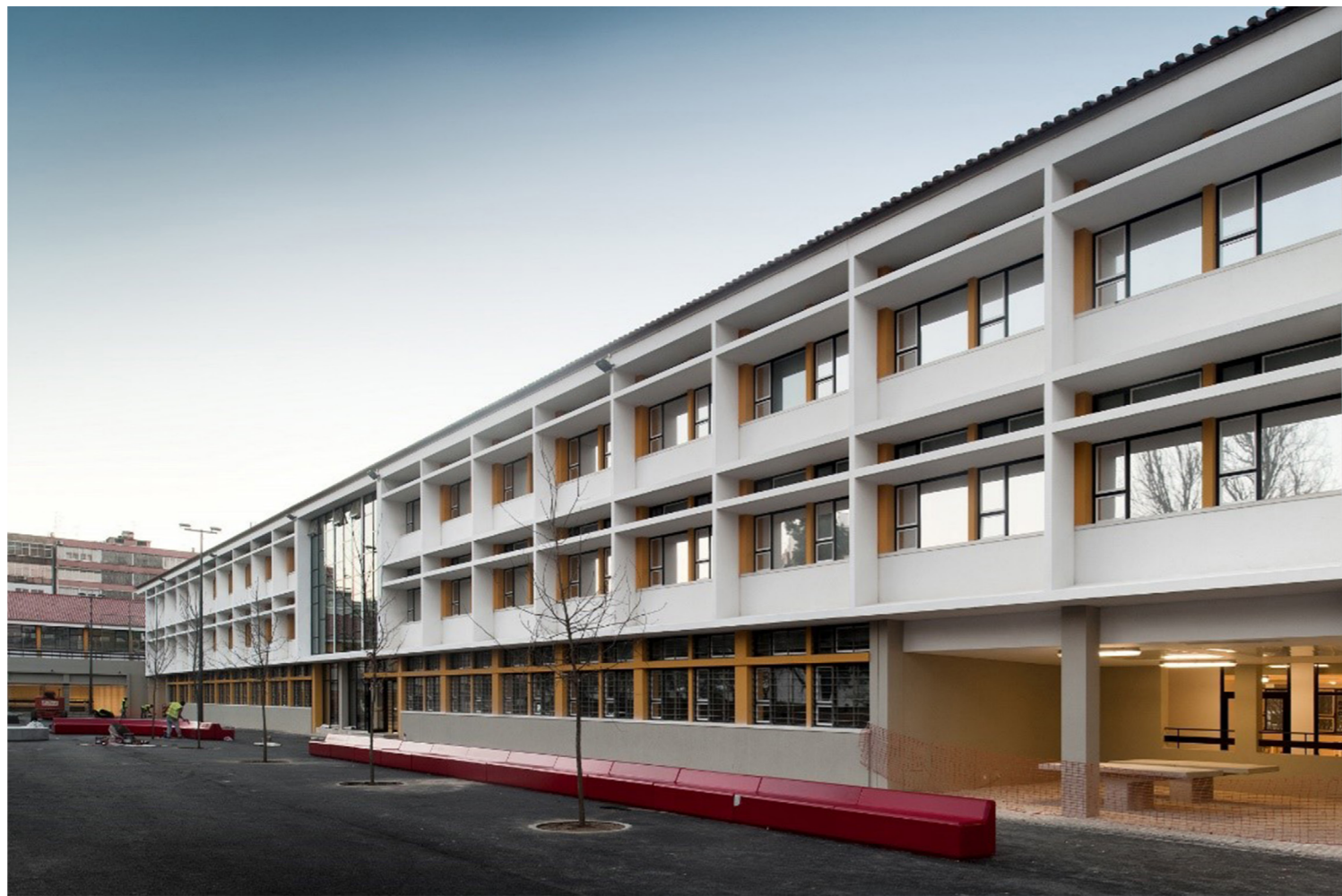
Fig. 4: RDLSS, Lisboa, Portugal, 2011. Rhythm of the structure visible in the existing building's façade after renovation. © FG+SG, 2010.
