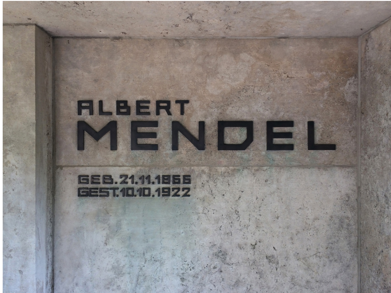
Fig. 8: Albert Mendel Grave, Jewish Cemetery Weissensee, Berlin, from Walter Gropius, 1923. Detail of the restored surfaces, joints and lettering. © Photo: Pedro Moreira, Archive Nedelykov Moreira Architekten, 2018.
