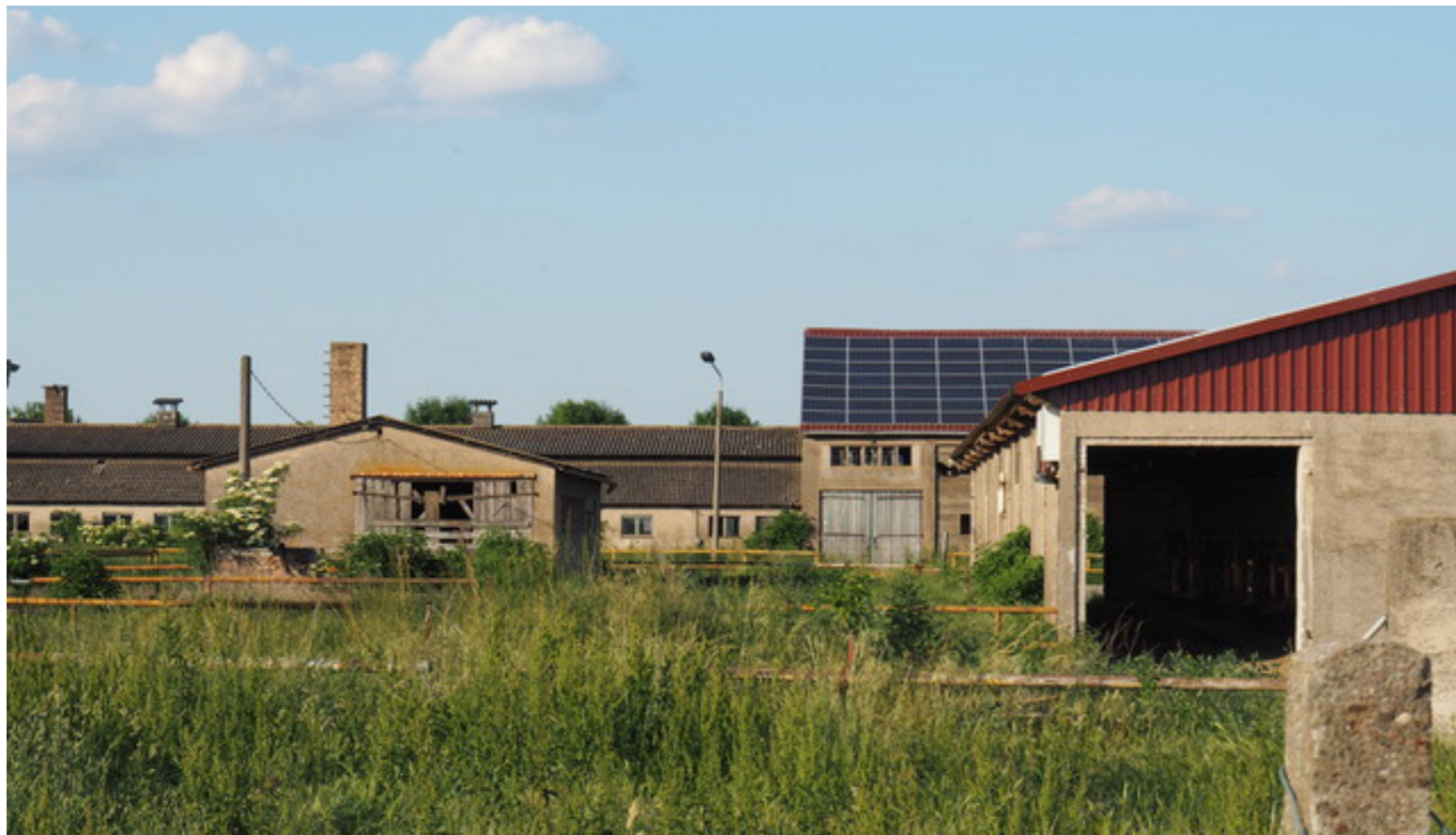
Fig. 2: Oderbruchhalle after renovation, 2018. Photo: © Emily Bereskin and Christoph Muth, 2018.
