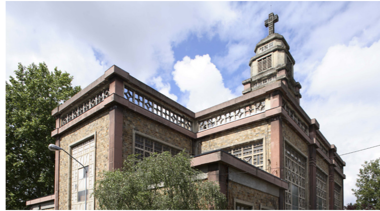
Fig. 6: Church of Saint-Suzanna, Schaarbeek (B), Eastern façade. © Photo: Oswald Pauwels Brugge, 2007.
