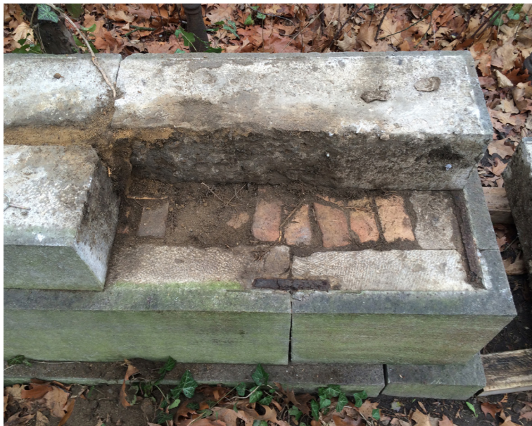
Fig. 3: Laura Perls Grave, Jewish Cemetery Weissensee, Berlin. Dismantling of the main volume with exposure of its core of bricks and earth, penetrated by ivy roots. © Photo: Pedro Moreira, Archive Nedelykov Moreira Architekten, 2015.
