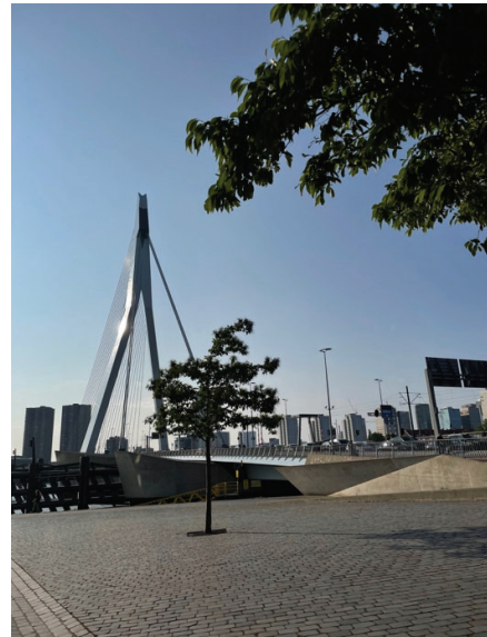
Erasmus-Brücke in Rotterdam
