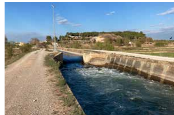
◀ Canal bringing the water to the agricultural areas
