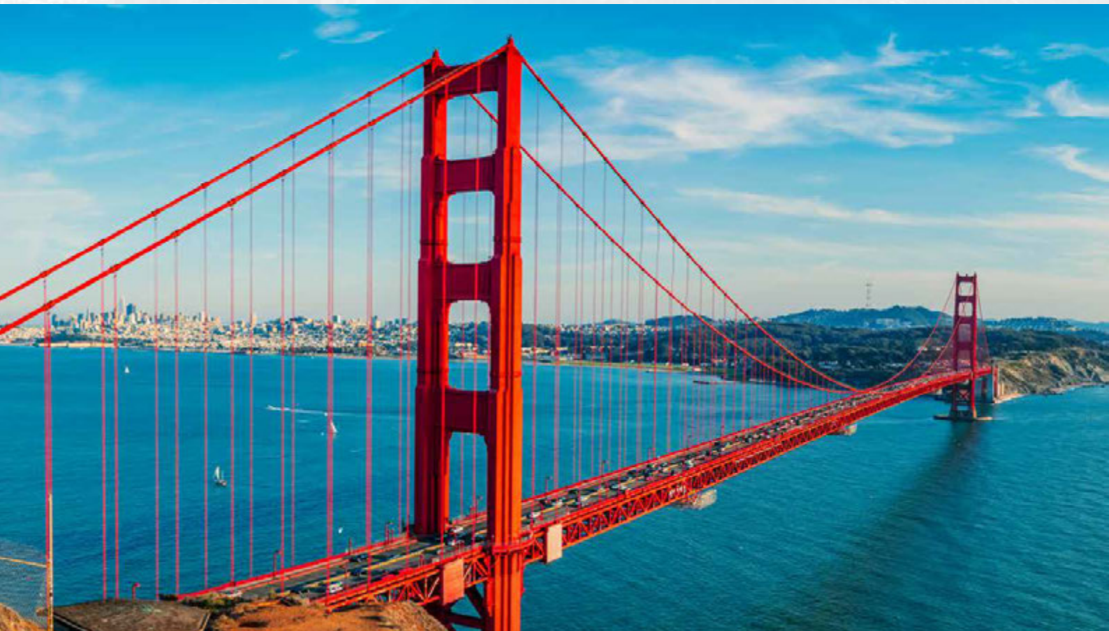
San Francisco, Golden Gate Bridge
